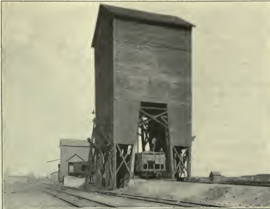
FIG. 667. FACILITIES TO BE ABANDONED. Locomotive coaling station of the Atchison, Topeka & Santa Fe Railway at Corwith Yard. This station has a storage capacity of 300 tons, and is operated by a gasoline engine. In the event of electrification, the station would be rendered worthless to the railroad. Beyond the coaling station is shown a sand house which could probably be utilized in its present location for furnishing sand to electric locomotives.
